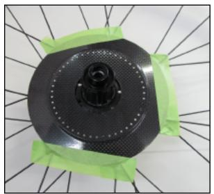
**Step 2 -** Center the disc on your hub and tape to the spokes so it cannot move around when lacing.
